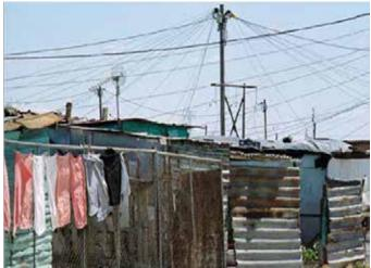
Figure 1: Indiscriminate Connection to an Electricity Supply Pole
