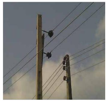
Figure 4 Broken cross poles
